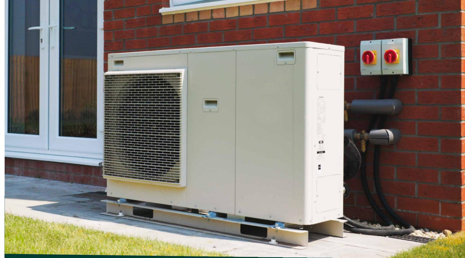
Your ASHP will normally be located under the window of the rear elevation, and the hot water cylinder will be located in a first floor cupboard. The cylinder will be between 150 and 300L in capacity, depending on the size of your home. Refer to your floorplans for the exact position in your house type.
