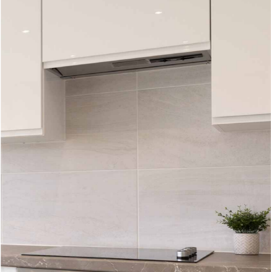
Tiling to underside of cooker hood
